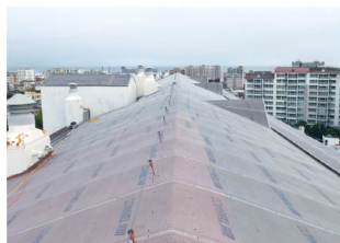
Mesh reinforcement
