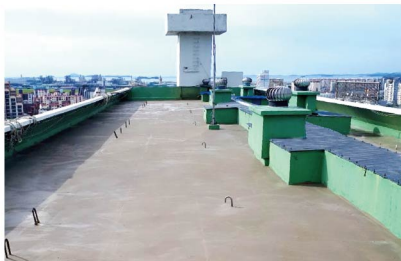
Rooftop waterproofing (Type A)
