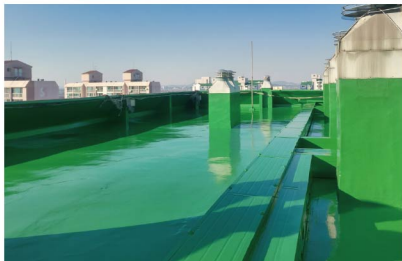
Rooftop waterproofing (Type B, C)
